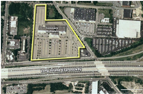
Aerial, Commack multiplex
